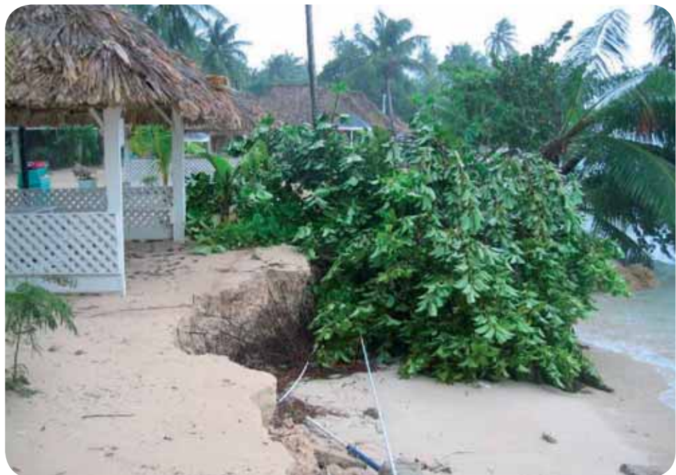
Hurricane Ivan Damage to Tourism Communications and Infrastructure, Tobago Credit: Dr Murray C Simpson
