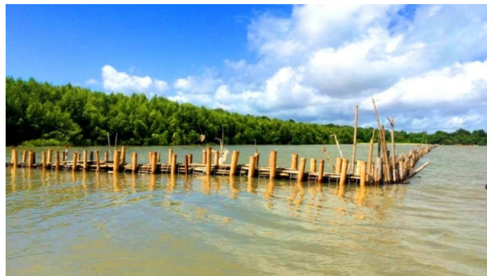
The semipermeable structures as sediment trap, Sawah Luhur village, Serang-Banten, West Java © Setyawati/MFF-Indonesia, 2016
