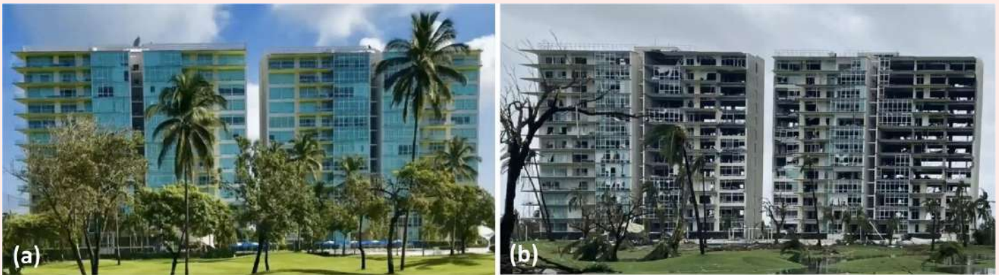
Fig. SB4.2. (a) Before and (b) after view of high-rise buildings and surrounding vegetation highlighting the severe wind impacts from Hurricane Otis in Acapulco, Mexico. (Photo credit: Parvez 2023.)
